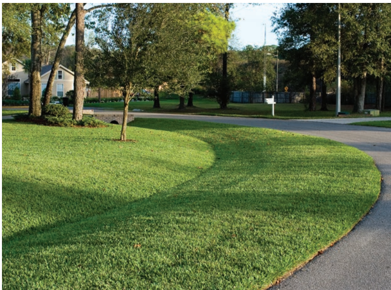
Stormwater swale
