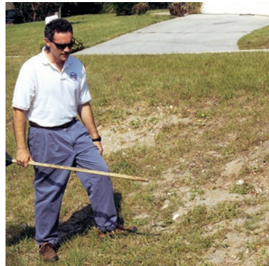
Repair eroded slopes.
