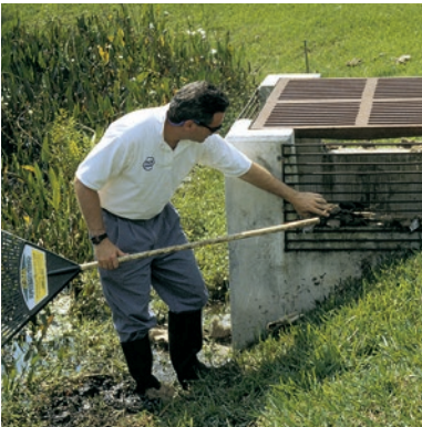
Keep inflow/outflow structures clean and clear of debris.
